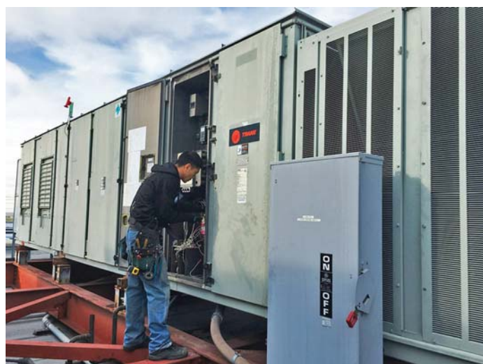
IoT sensors being installed to monitor a 90-ton rooftop HVAC unit via an Intel BMP gateway. (Photo courtesy CANDI)
